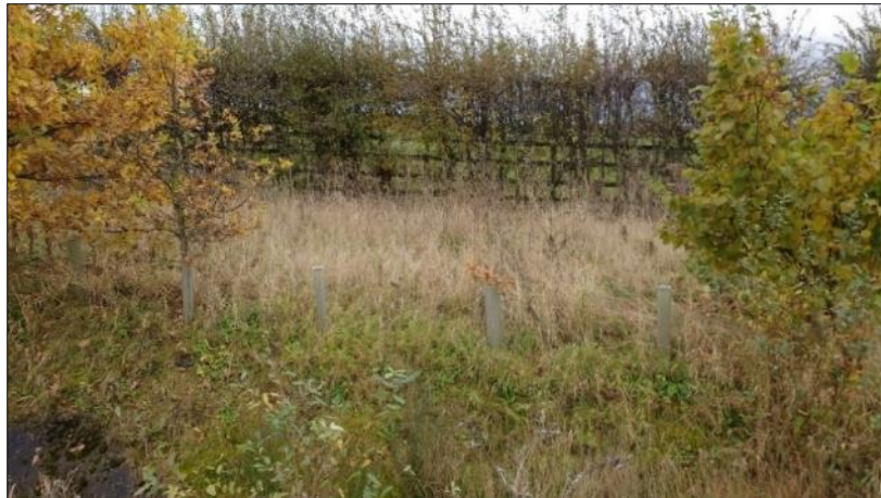
Figure 9.4: Planting to the south of the carriageway fails to compensate for loss of mature trees and hedgerows in an area formerly of Great Landscape Value where the road vegetation was a 'significant landscape feature'
