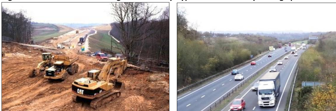
Figure 7.7: Excavation of cuttings for Newbury Bypass and a close-by vantage point in 2016
