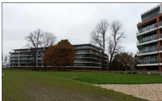
Figure 7.10 Development of flats along north side of Newbury Racecourse
