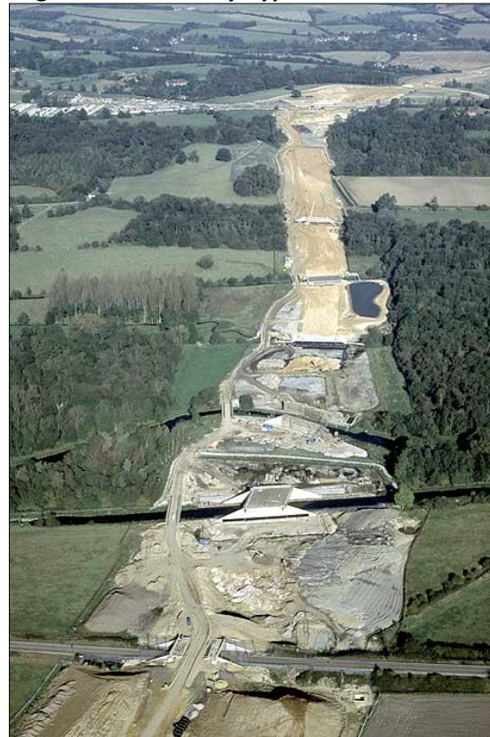
Figure 1.2: Newbury Bypass construction
