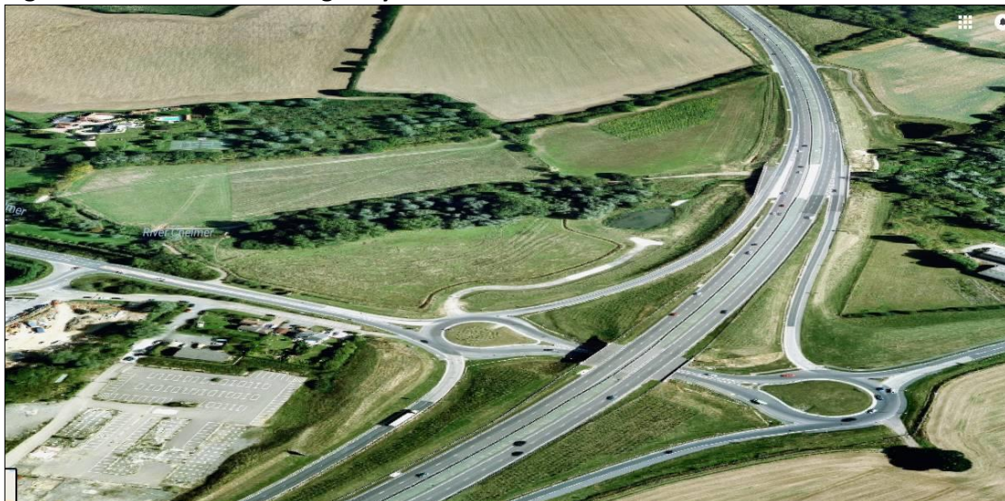
Figure 10.2: A120 dual carriageway south of Great Dunmow
